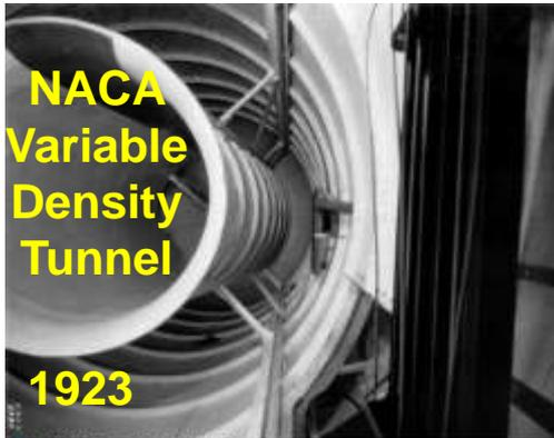
Variable Density Tunnel - Wind Tunnel #2
